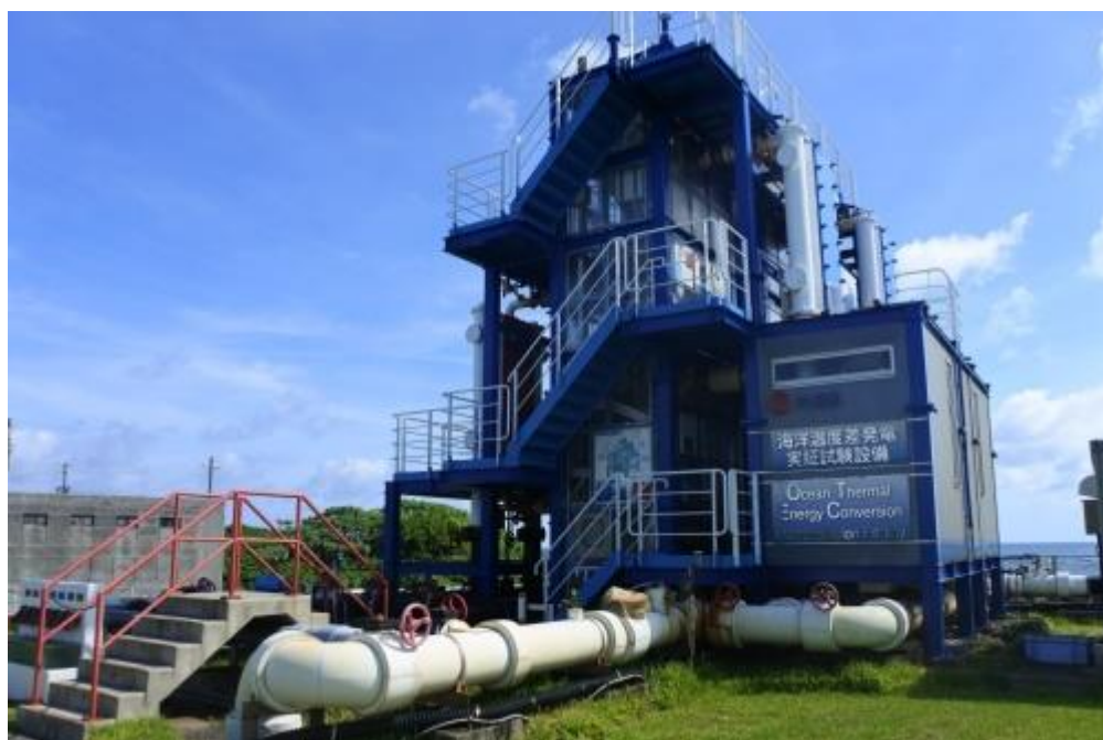
Figure 1 • Ocean-thermal energy conversion demonstration facility operating in Kumejima, Okinawa Prefecture
