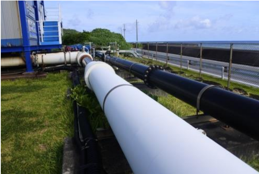
Figure 4 • White pipe through which deep seawater of 8 to 9°C is running, and black pipe through which surface seawater of 26°C is flowing
