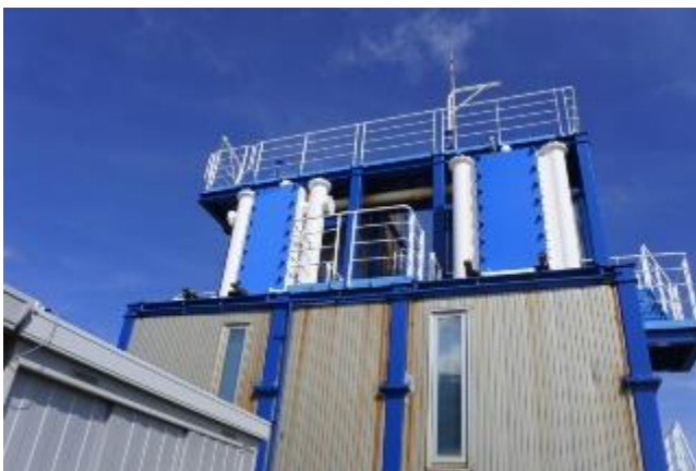
Figure 5 • Two blue installations that are plate-like in shape contain plate-type heat exchangers
